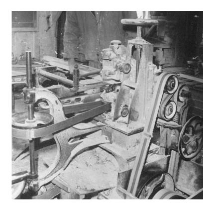
A rip saw, band saw, thickness planer, boring machine, and sticker for specialty mouldings and trims, were all belt-driven at speeds ranging from 1,200 to 2,500 rpm. Other machines from the same period, notably a sander and a tenoner, have also survived but are not currently in use, possibly because such antiquated equipment has been described by one unsettled operator as not only unsafe, but also scary.
