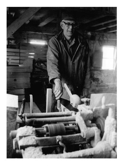
The machine operator (in this case long-time Mundell Lumber employee Stan Howlett, photographed in 1975) can engage or disengage a specific machine from the line shafting by moving a wooden lever which slides the moving belt from an idler pulley onto a drive pulley located beside it on the same countershaft.
